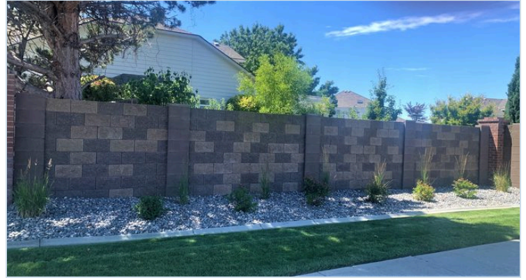
After — the new masonry wall and landscaping.
